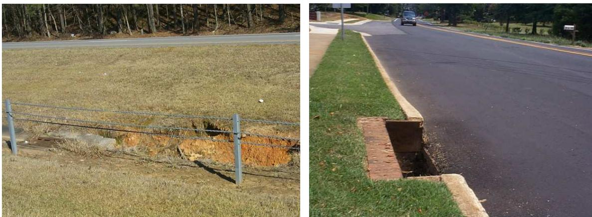
**Figure 3.11 – Inlets Damaged**
