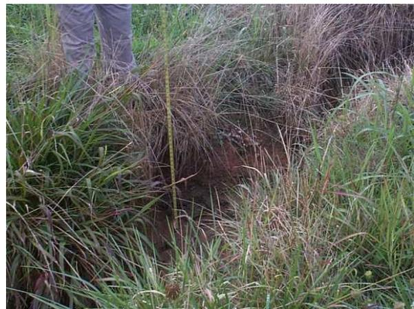
**Figure 3.4 – Lateral Ditches Eroded**
