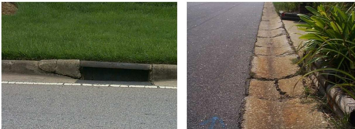
**Figure 3.9 – Gutters Damaged**
