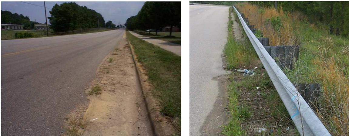
**Figure 3.8 – Gutters Blocked**
