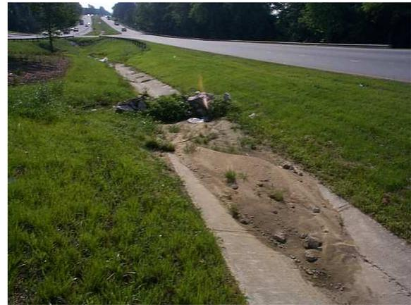
**Figure 3.3 – Lateral Ditches Blocked**
