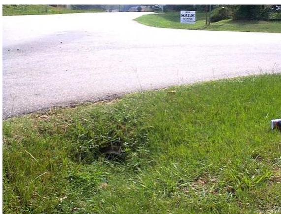
**Figure 3.6 – Crossline Pipes Blocked**
