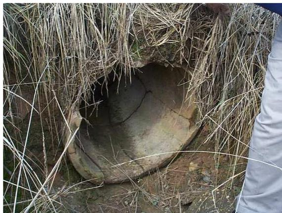
**Figure 3.7 – Crossline Pipes Damaged**
